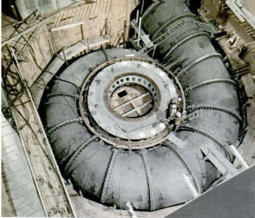
Shail-like scroll case feeds water to turbine waterwheel at 53 miles an hour
